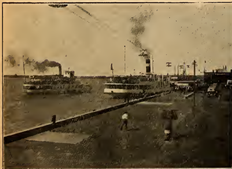
AUTOMOBILE FERRY WHARF, SARNIA
